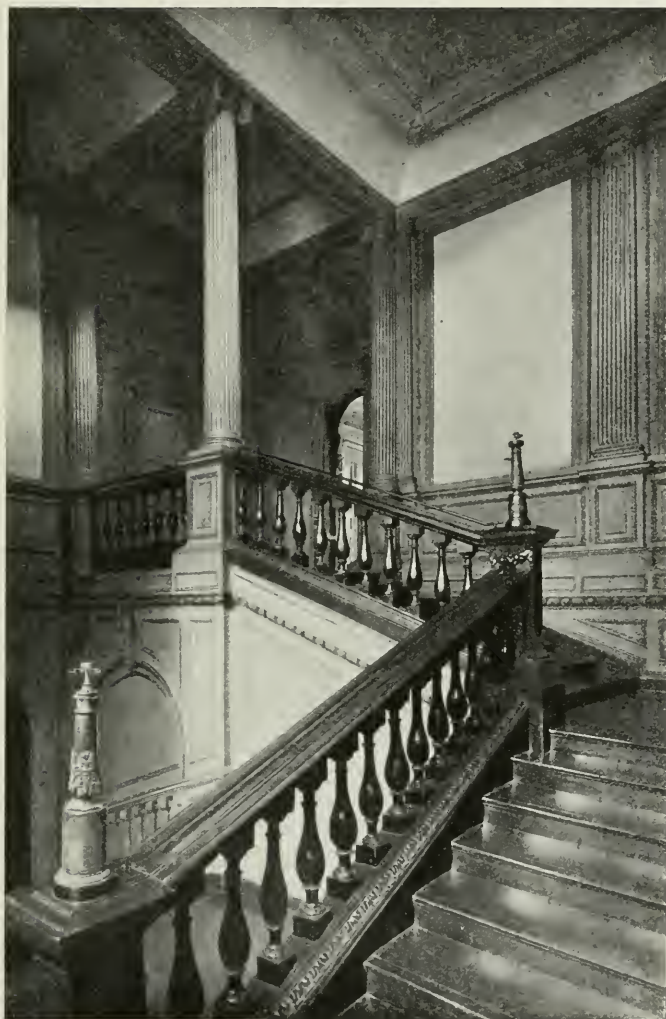
171. Staircase, Ashburnham House, Westminster.
